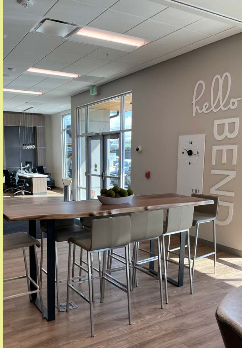
Bend office LED lighting
